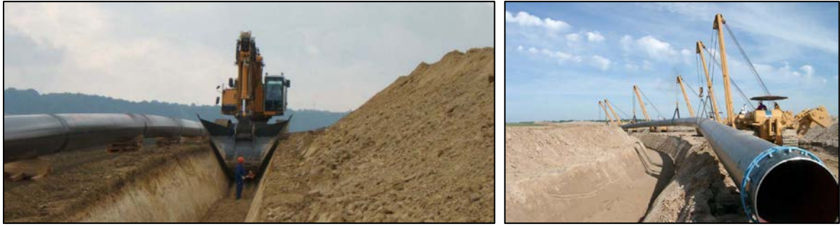
Figure 6-21 Onshore pipeline trench excavation (left) and the pipeline being lowered into the trench.
