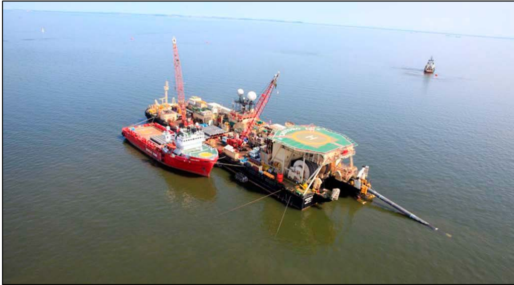
Figure 6-22 Typical shallow water lay barge (with anchor tug and pipe transportation vessel).
