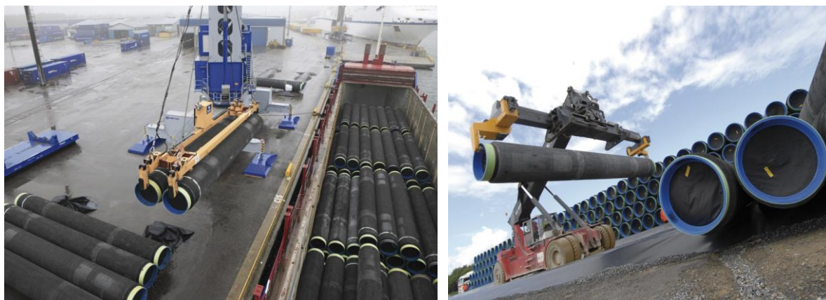
Figure 6-13 Offshore pipe supply
