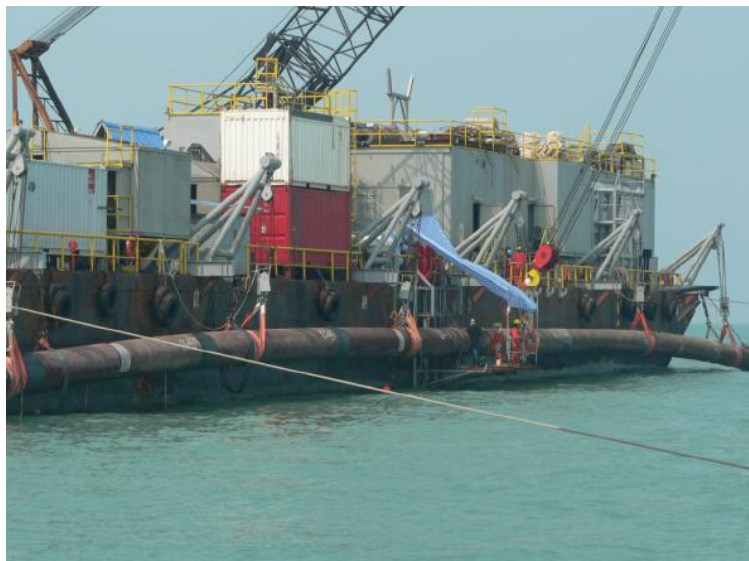
Figure 6-22 Typical pipeline configuration during AWTI
