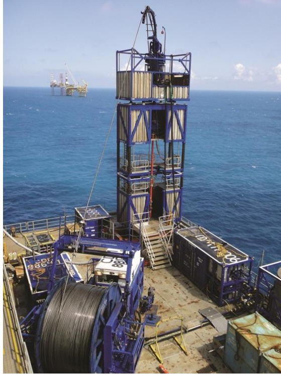
Figure D-5 Well intervention at Halfdan, 2012
