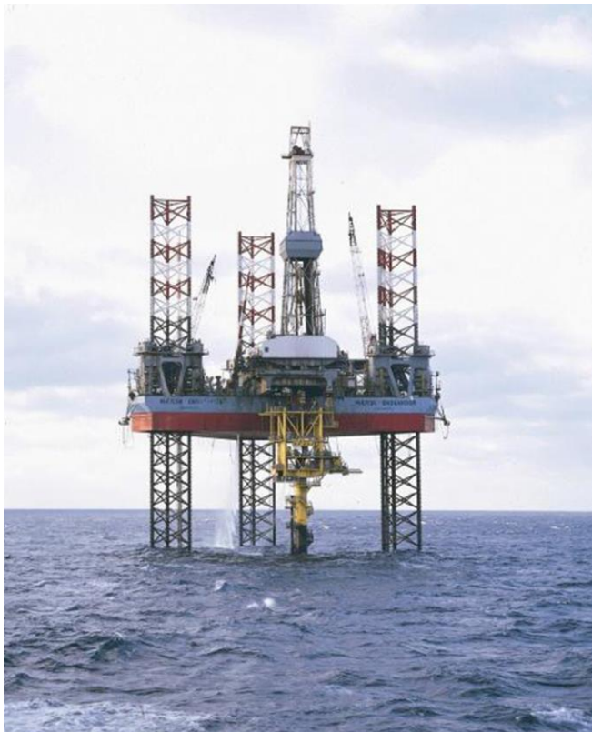
Figure D-1 Typical jack-up drilling rig (Maersk Endeavour), here situated at the Kraka STAR platform
