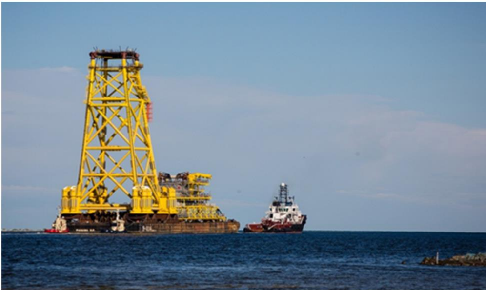
Figure B-4 Tyra SE-B facilities (jackets, top side and bridge) – tugged to location in 2014
