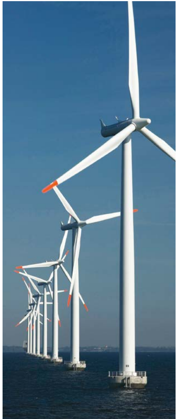
Nysted Offshore Wind Farm. PHOTO: NYSTED OFFSHORE WIND FARM
