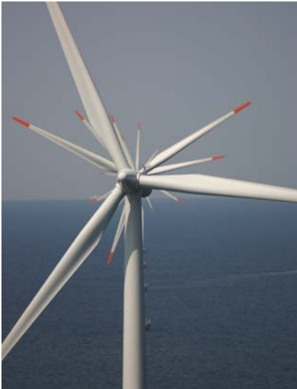
Nysted offshore wind farm at hub height.
