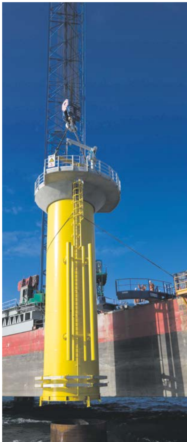
Preparation of monopile foundation at Horns Rev 2.
