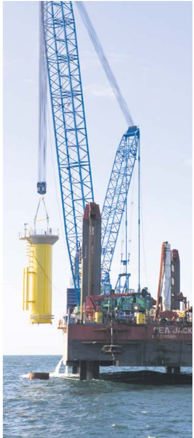
Construction of monopile foundations at Horns Rev 2.
