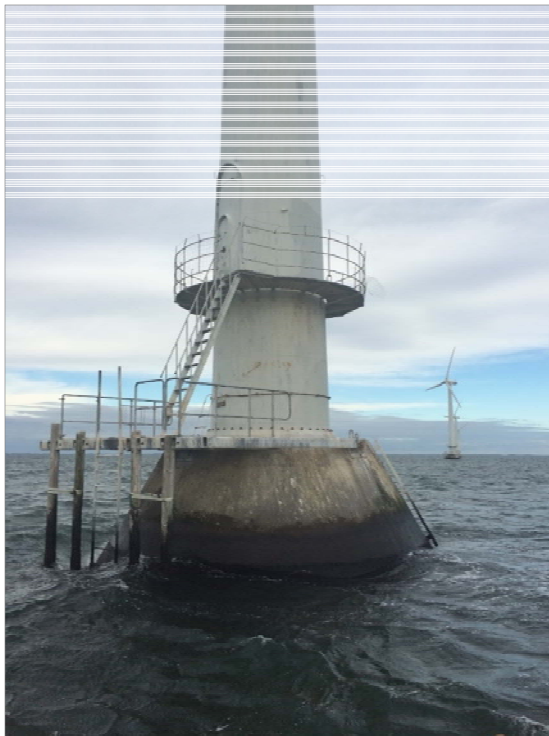
Figur 3: Gravitationsfundament i Vindeby
