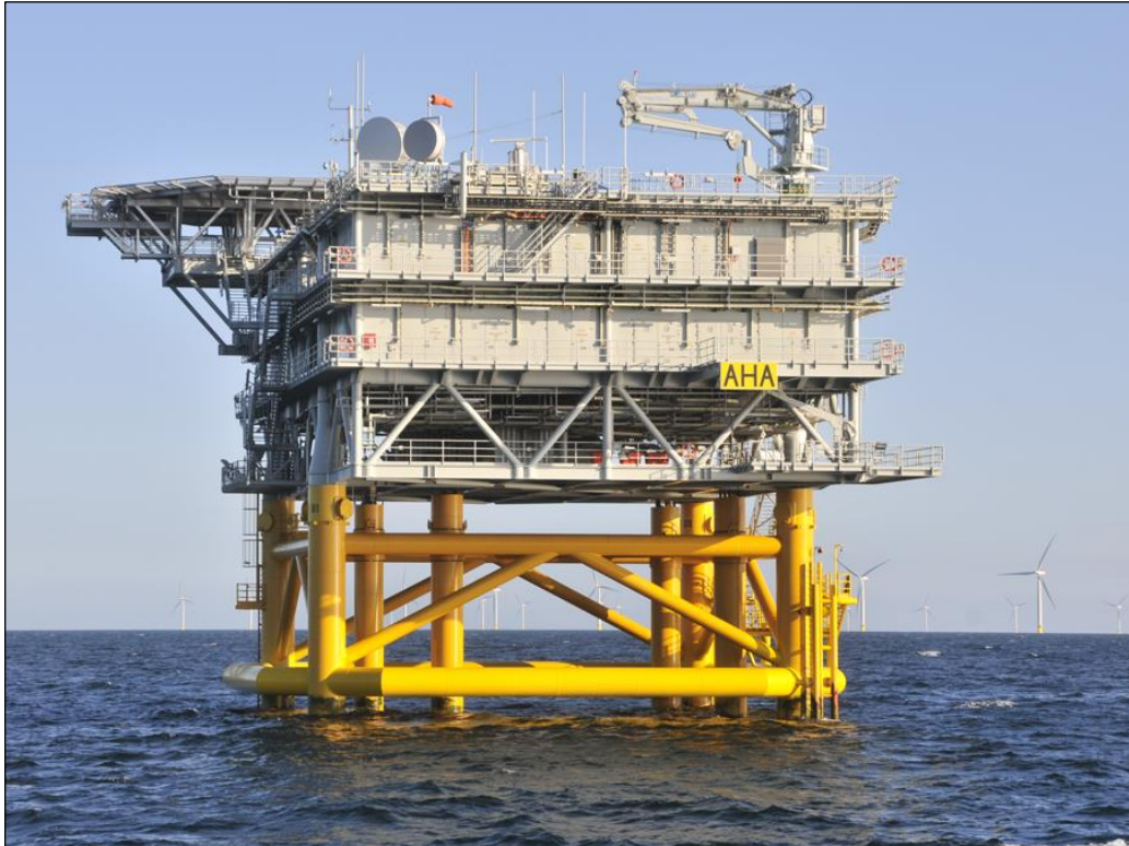
Figure 5-3. The Substation with the helicopter deck (top left side and 23 m above sea level) which was used for observations and rangefinder tracking of migrating raptors. Photo Lars Maltha Rasmussen.
