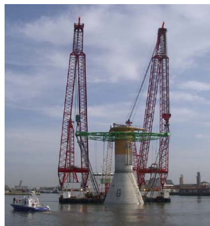
Figure 4-10: Transport to site of GBS. Thornton Bank (Courtesy: Cowi)
