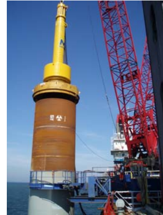
Figure 4-6: Driving of Monopile Burbo Banks (Courtesy: MT Højgaard)
