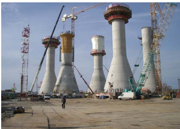
Figure 4-9: GBS under construction. Thornton Bank (Courtesy: Cowi)
