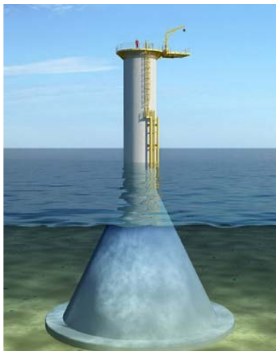
Figure 4-7: Typical GBS cone foundation (Courtesy: Ramboll)
