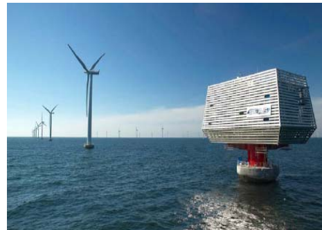
Figure 4-13: Transformer Station. Rødsand (Courtesy: SEAS)
