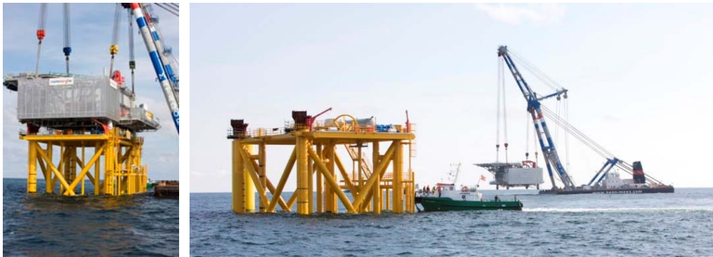
Figure 4-14 and 4-15: Installation of transformer station. Horns Rev I. (Courtesy: ENDK)
