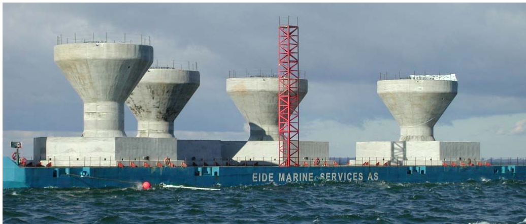
Figure 4-8: Transport to site of GBS. Rødsand (Courtesy: Aarsleff)
