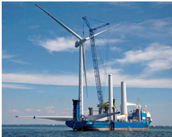
Figure 4-4 Installation of tower and nacelle Lillgrund (Courtesy: A2SEA)
