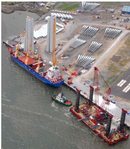
Figure 4-3 Port facilities Burbo Banks (Courtesy: Siemens)
