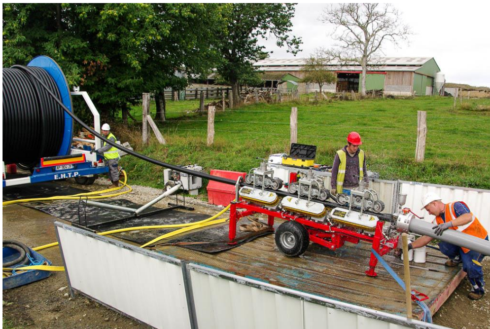
Watucab machine installing cable
