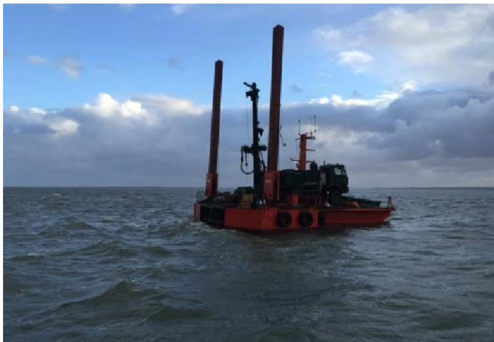
Barge with drilling rig on site, September 2016
