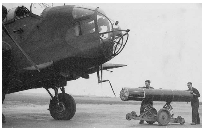
Figure 3.2 - Hampden being loaded with British ground mine
