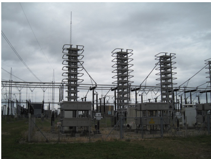
Figur 3.7: Filterfelt
