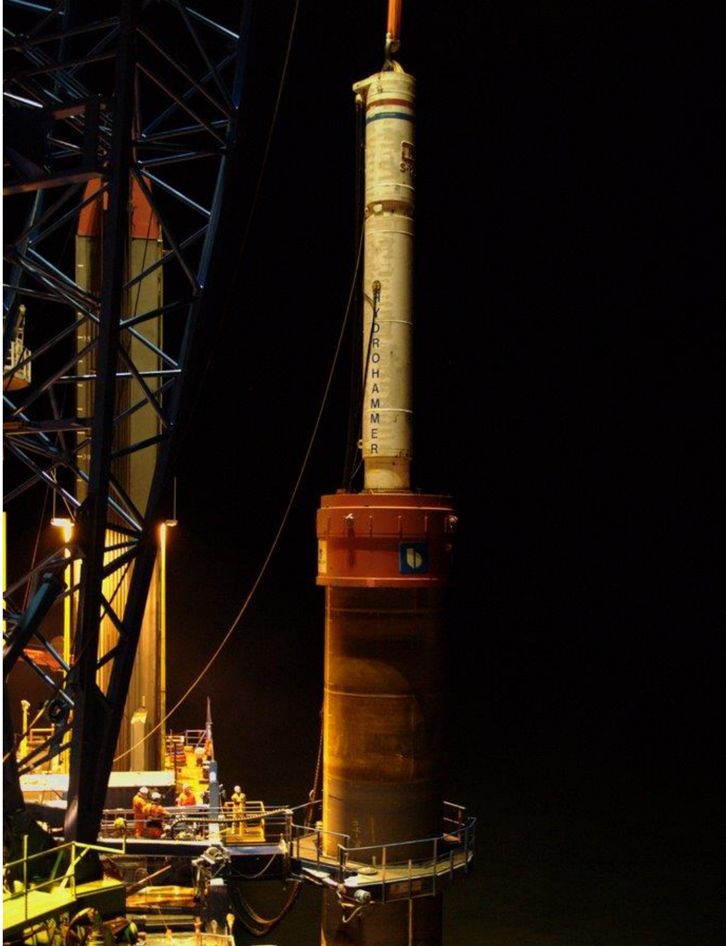
Piling of monopiles at Horns Rev 2 Offshore Wind Farm
