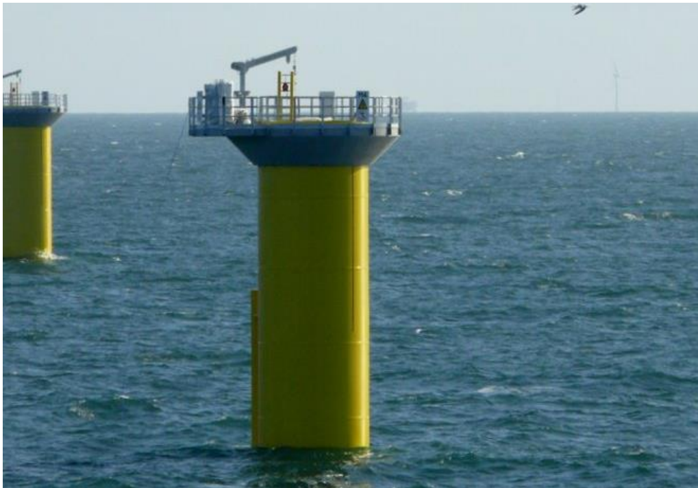
Monopile foundation – Horns Rev 2
