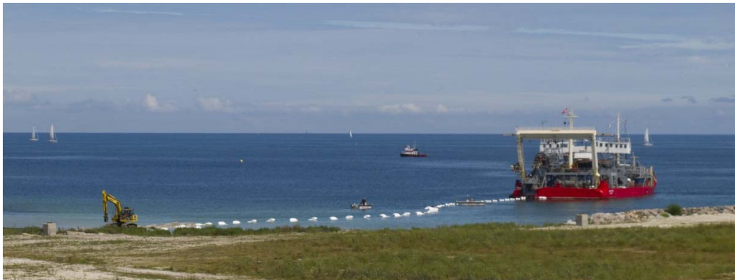
Cable laying vessel near shore
