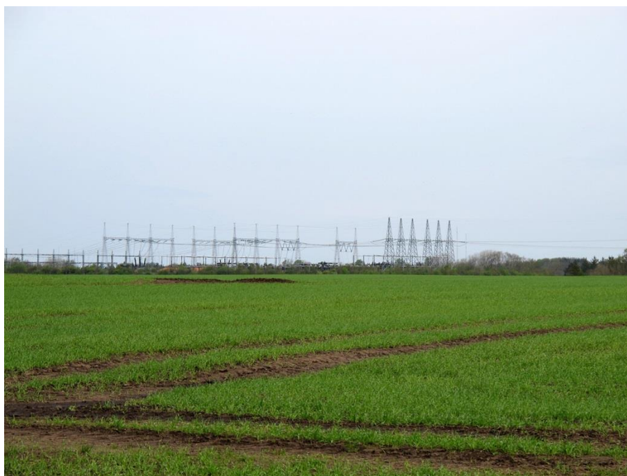
Transformerstation set fra Endrup
