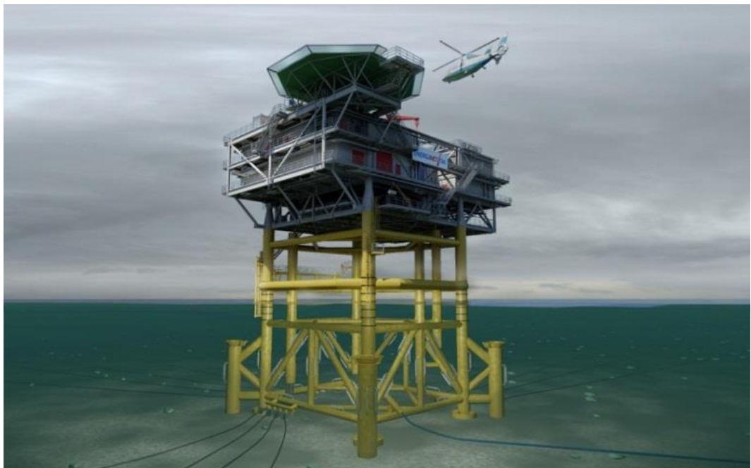
Figur 2-6. Jacketfundament.
