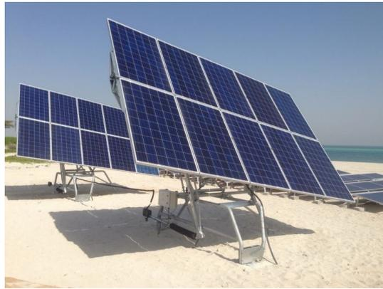
Figure 6 A Helioslite 1.5 tracking system (Ref. 13).
