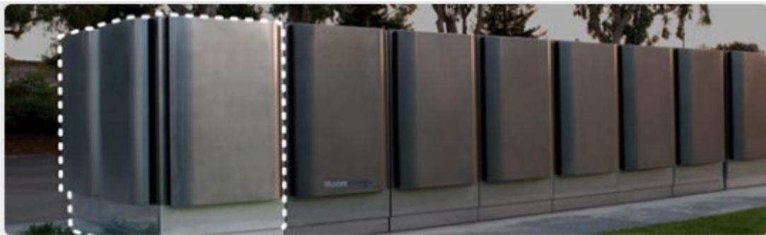
Figure 4: BloomEnergy SOFC system. The dashed region corresponds to the 250 kW<sub>e</sub> unit [1].
