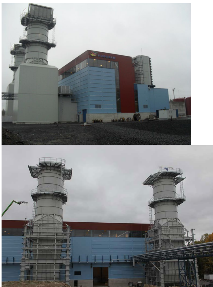
Figure 3 Forssa Power plant commissioned for Fingrid [17].
