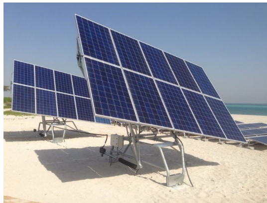
Figure 6 A Helioslite 1.5 tracking system (Ref. 13).
