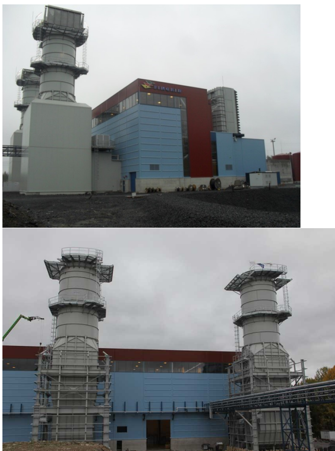
Figure 3 Forssa Power plant commissioned for Fingrid [17].
