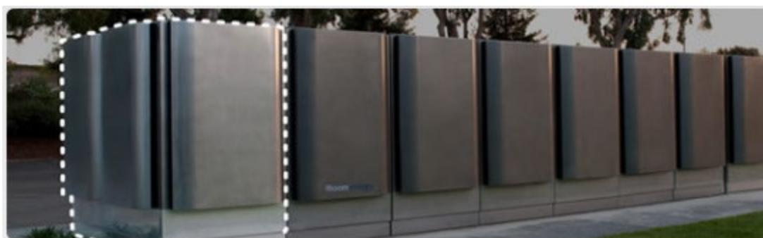
Figure 4: BloomEnergy SOFC system. The dashed region corresponds to ine 250 kW<sub>e</sub> unit [1].
