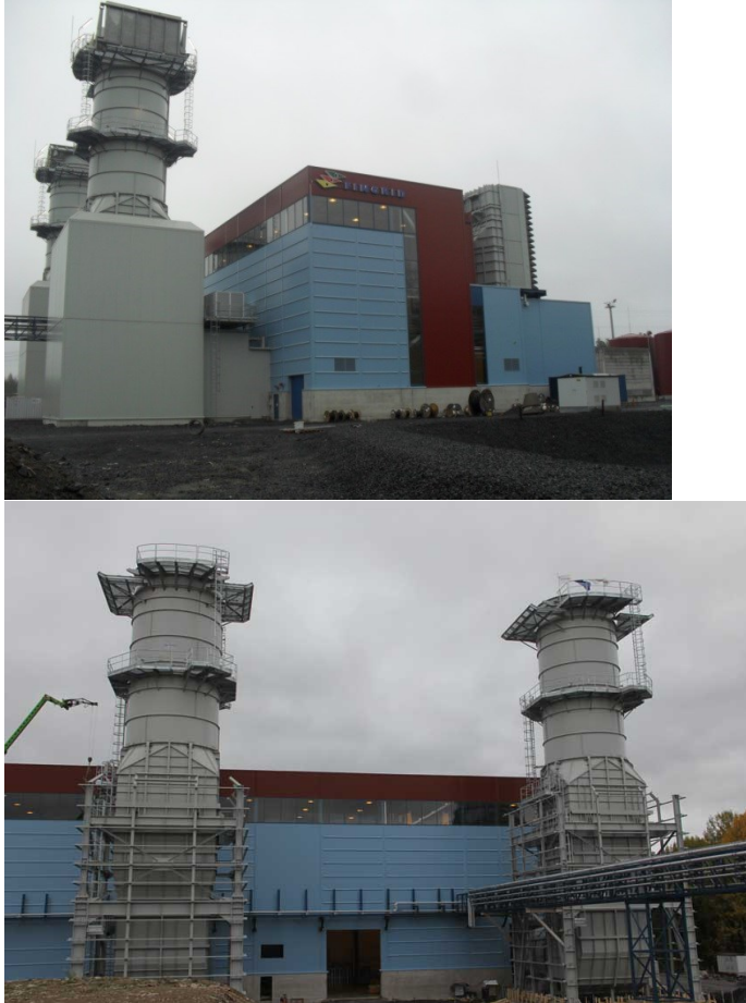
Figure 3 Forssa Power plant commissioned for Fingrid [17].
