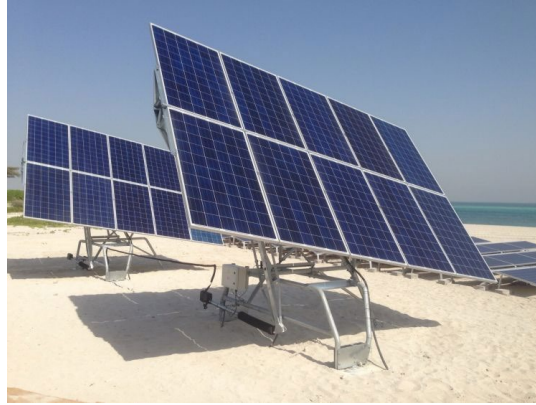
Figure 29 A Helioslite 1.5 tracking system (Ref. 13).
