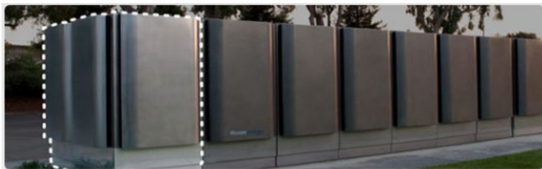
Figure 4: BloomEnergy SOFC system. The dashed region corresponds to ine 250 kW e unit [1].
