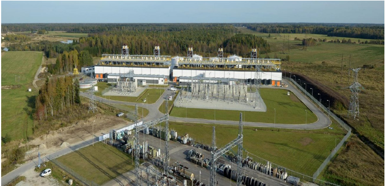
Figure 3 Kiisa emergency reserve power plant (ERPP) in Estonia [14].
