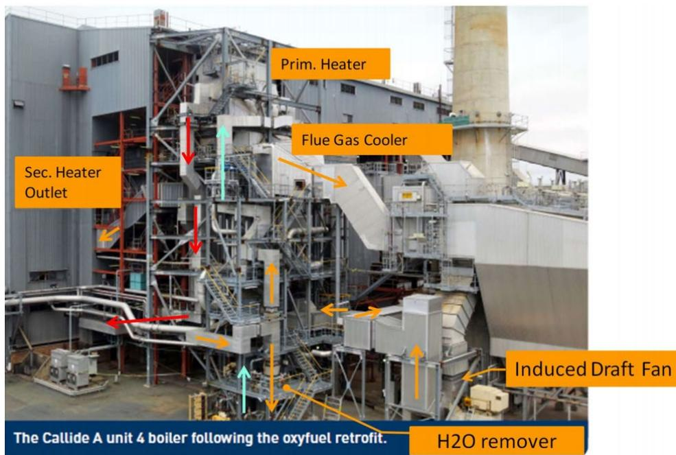
Figure iii-10 Photo of Callide Oxy-fuel boiler from [52] showing retrofit paths (red) and flue gas flow directions (yellow).
