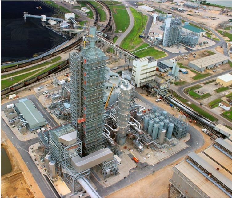
**Figure ii-5. Petra Nova amine CC plant retrofitted to a slip stream of flue gas (equivalent to 240 MWe) from the WA Pariash unit 8 coal-fired power plant. Source: <https://www.nrg.com/case-studies/petra-nova.html>**
