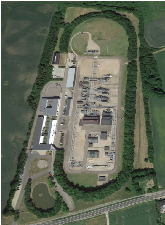
Figure 0-9: Stenlille gas storage [9]
