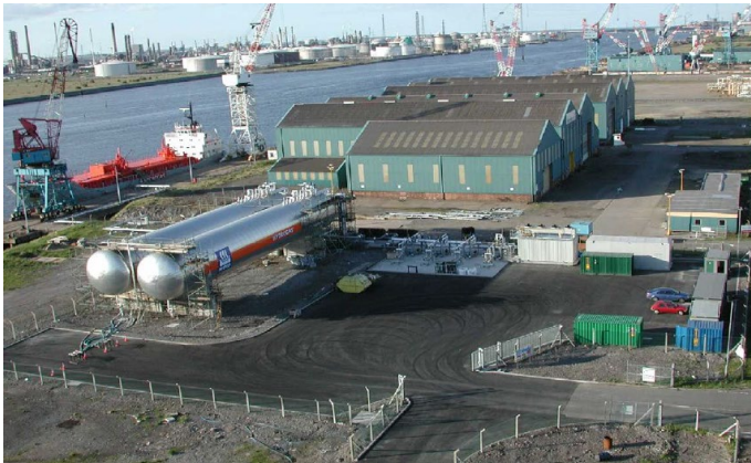
Figure 10. Liquid CO 2 import terminal with truck filling bays operated by Yara (now Nippon Gases Norway). [7]
