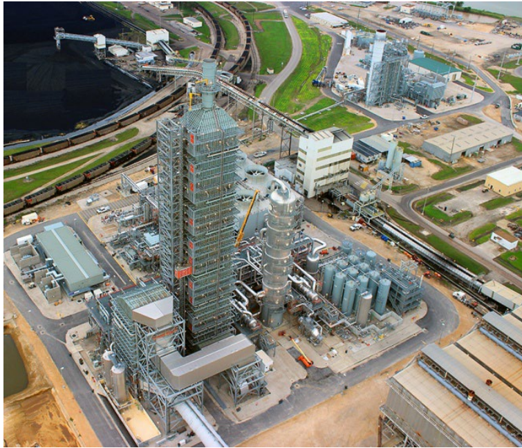
Figure 5. Petra Nova amine CC plant retrofitted to a slip stream of flue gas (equivalent to 240 MWe) from the WA Parish unit 8 coal-fired power plant. Source: https://www.nrg.com/case-studies/petra-nova.html
