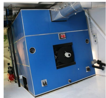
Figure 22: 250 kW pellet boiler for large buildings from LIN-KA [16]
