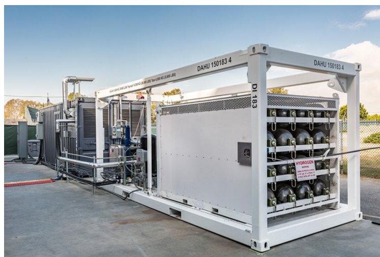
Figure 2: SOEC hydrogen plant from Sunfire [11].
