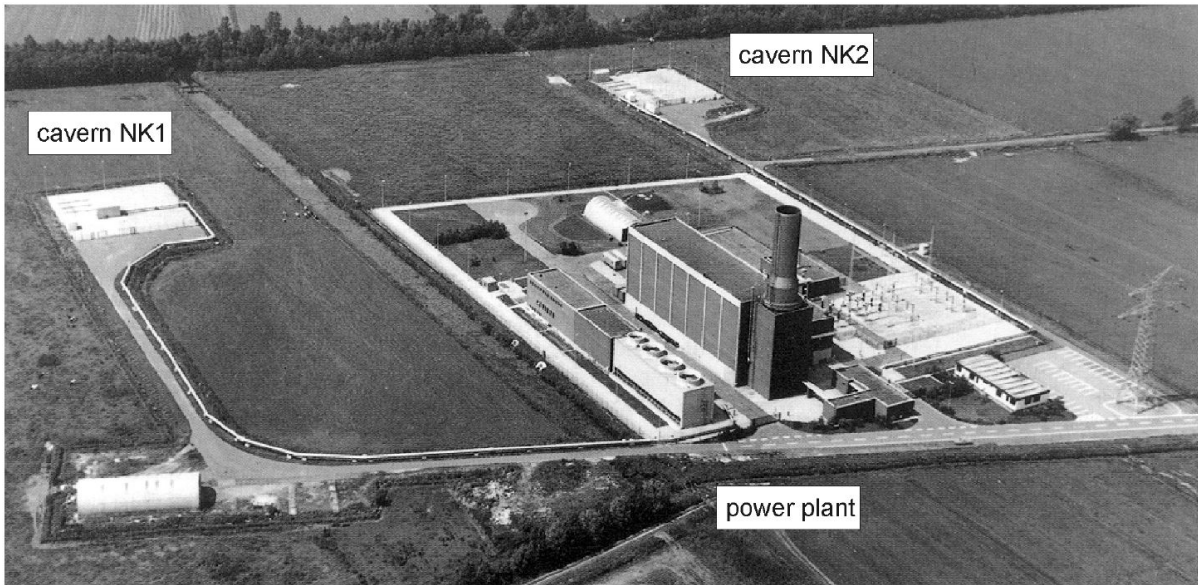
Figure 6: Aerial photo of the Huntorf facility [12] .
