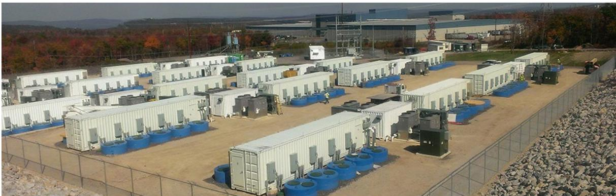
**Figure 5: Photo of Beacon Power flywheel installation in commercial operation in PJM, Hazle, Pennsylvania. The plant includes 200 flywheel modules lowered into the ground (5 on each side of a container). The plant currently provides 20 MW of frequency regulation service to PJM and reached full commercial operation in July 2014 [6].**
