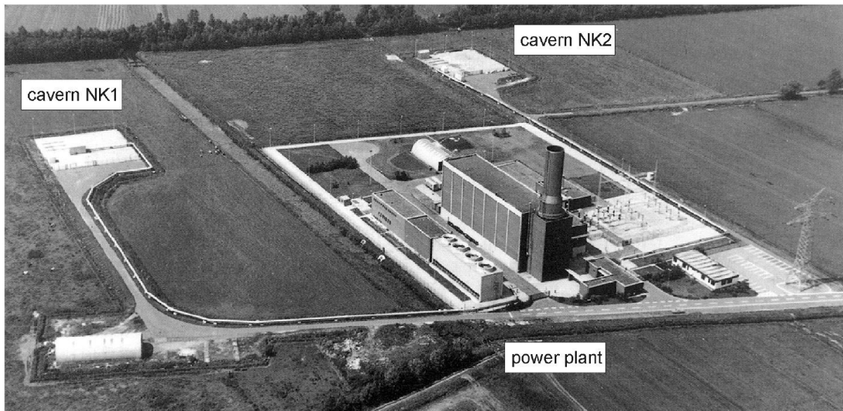
Figure 6: Aerial photo of the Huntorf facility [12] .
