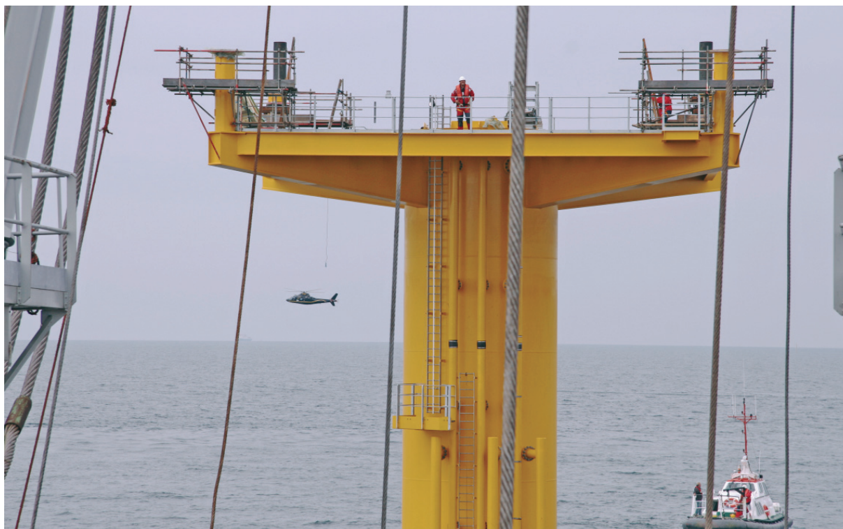
Figur 5.4 Installation af offshore substation (Barrow, 2006).
