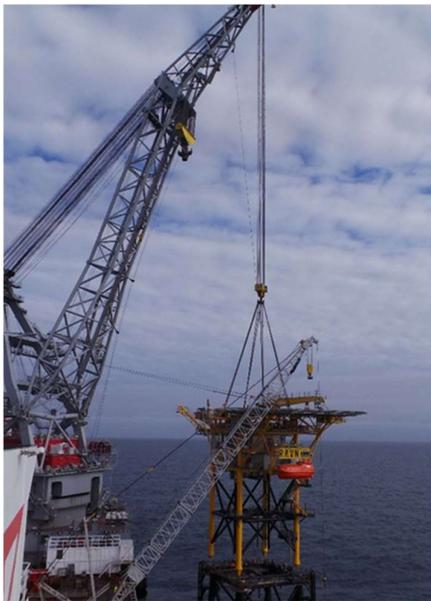
Figure 6-13 Lifting of Topside (example from erecting).
