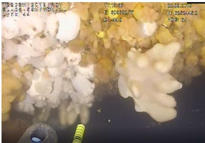
Figure 6-15 Example of marine growth on jacket.
