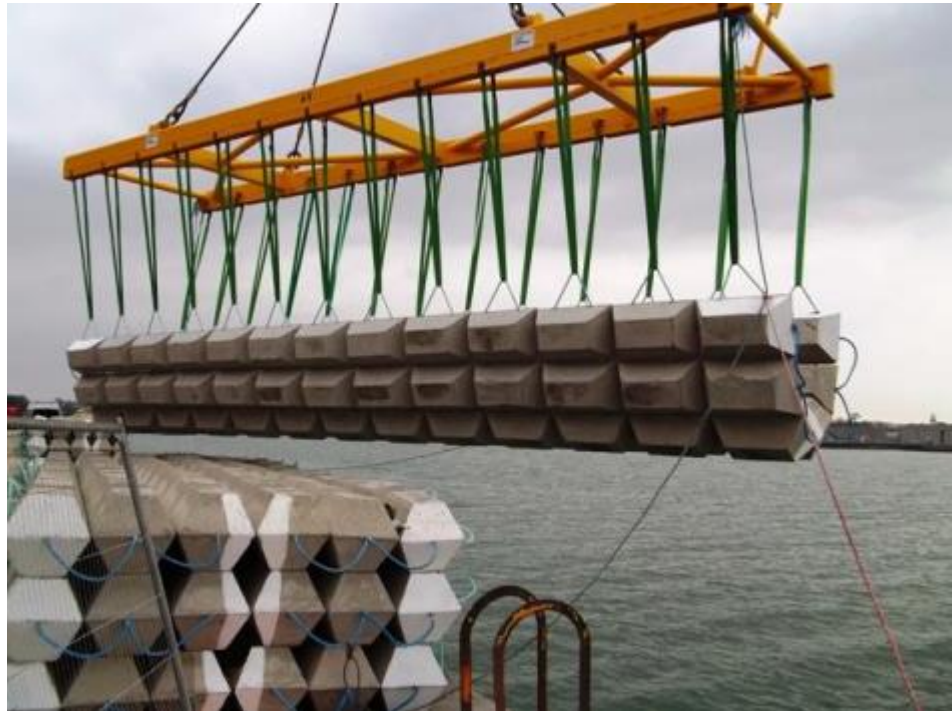
Figure 5.4: Laying of concrete mattresses. 16
