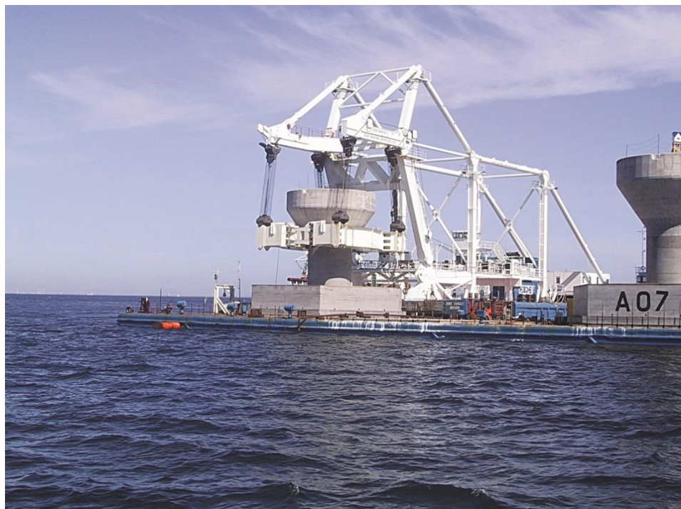
Figure 3.7: GBS installation from a flat top barge using a floating crane.
