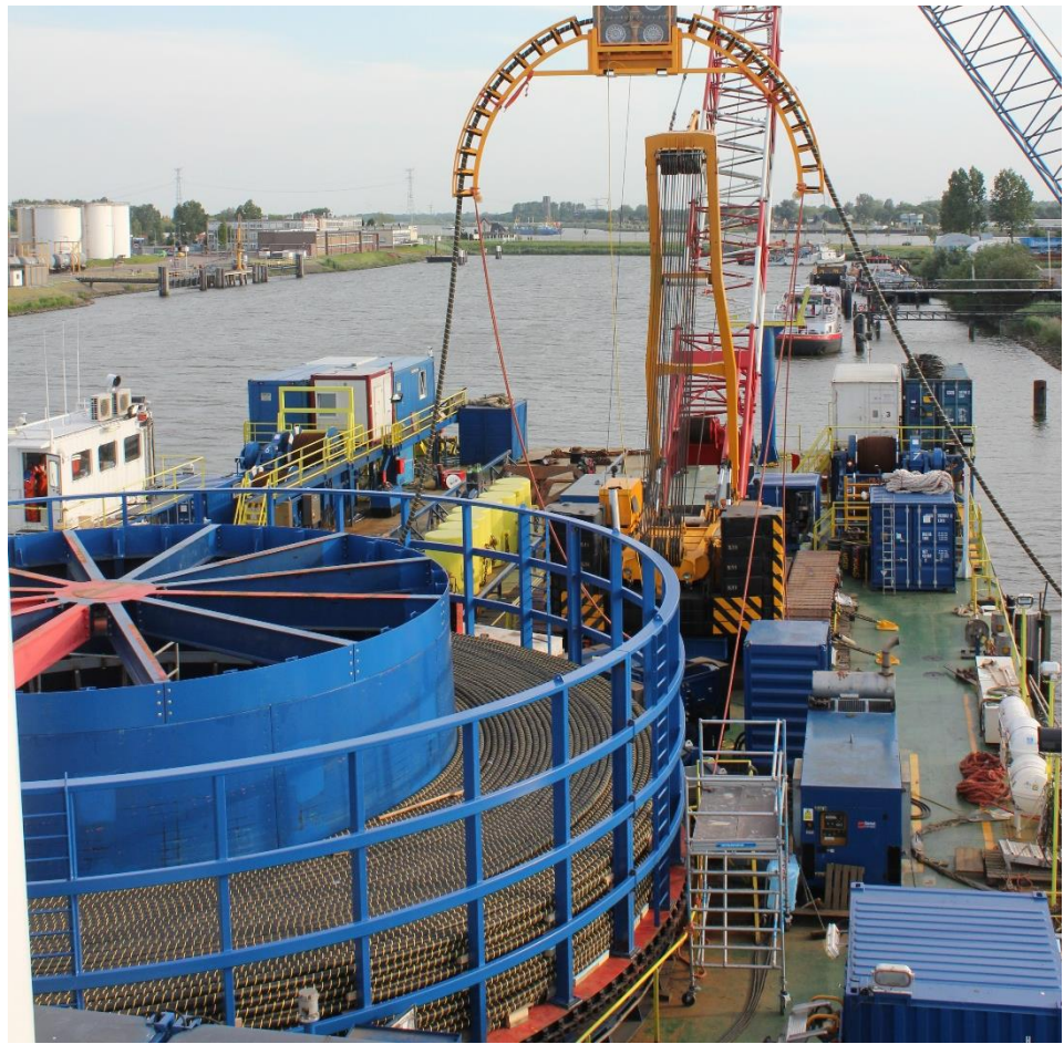
Figure 5.1: Cable in turn table aboard cable laying vessel.
