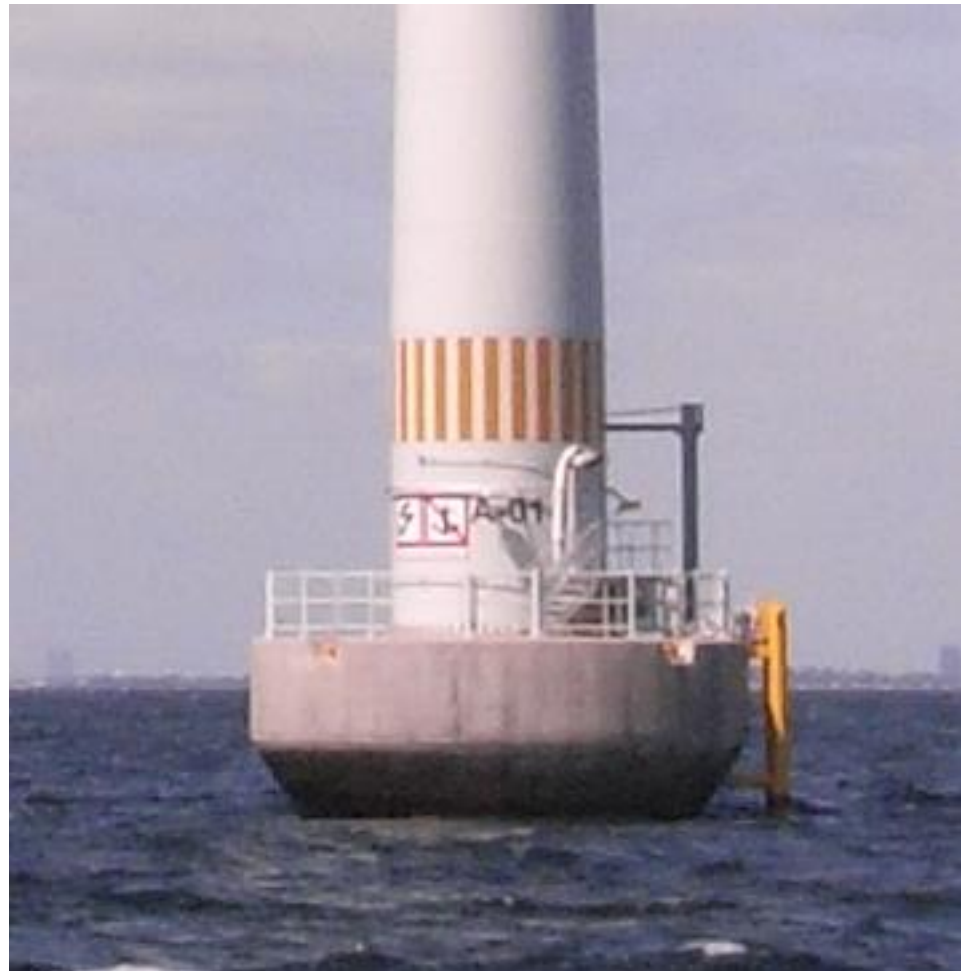
Figure 3.5: GBS foundation with ice deflection cone.
