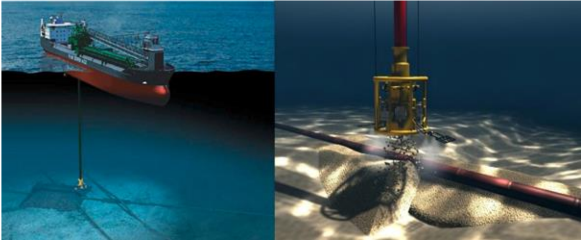
Figure 6-19 Rock placement on the seabed through a fall-pipe.
