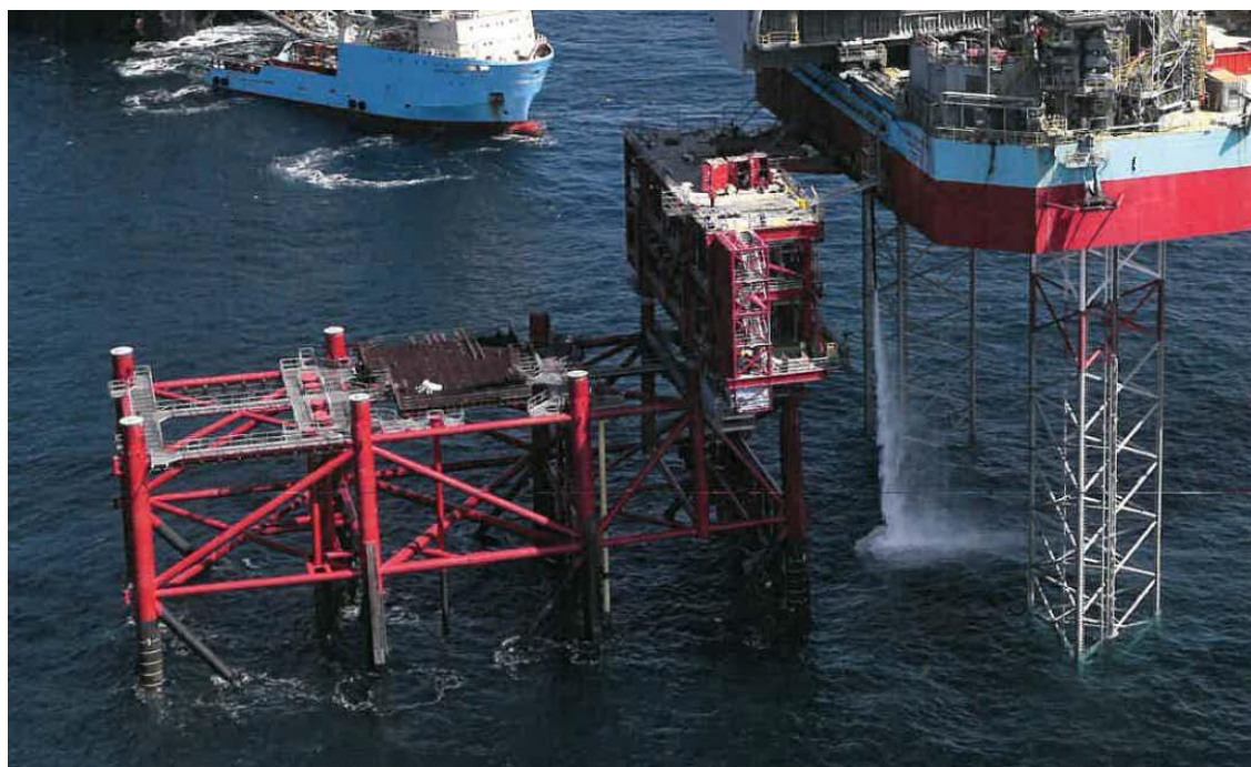
Figure 2-5 Hejre field well drilling by Mærsk Resolve, summer 2015
