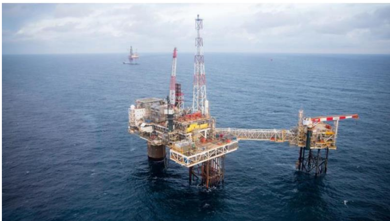
Figure 5-5 South Arne and well head platform East.
