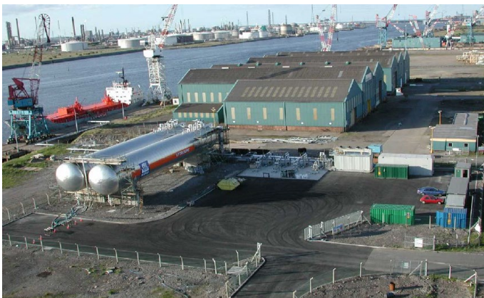
Figure 10. Liquid CO 2 import terminal with truck filling bays operated by Yara (now Nippon Gases Norway). [7]
