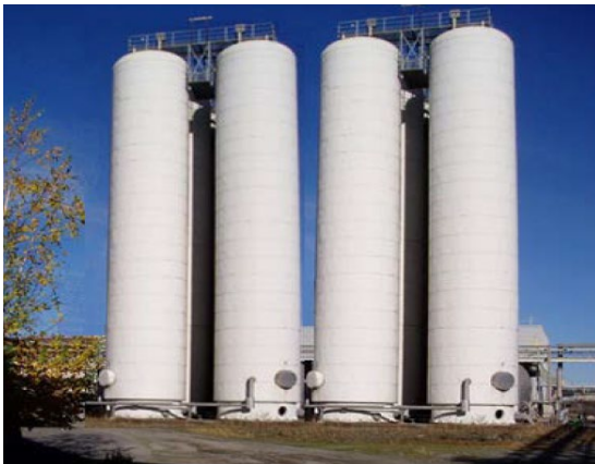
Figure 9. Storage for 3300 tons liquid CO 2 at Yara's ammonia plant in Porsgrunn, Norway in conjunction with CO 2 export terminal (now operated by Nippon Gases Norway) [7]
