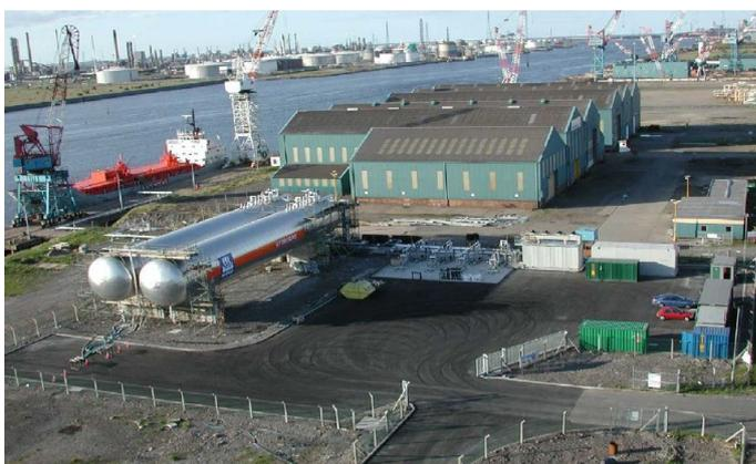
**Figure 10. Liquid CO<sub>2</sub> import terminal with truck filling bays operated by Yara (now Nippon Gases Norway). [7]**
