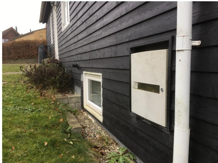
**Figure 4** Cupboard containing pressure regulator and flowmeter mounted outside a private house.
