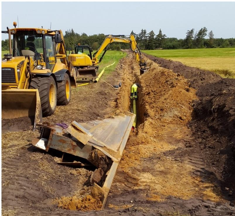
**Figure 3 Routing of gasline with distribution pipe. Source: HMN Gasnet.**
