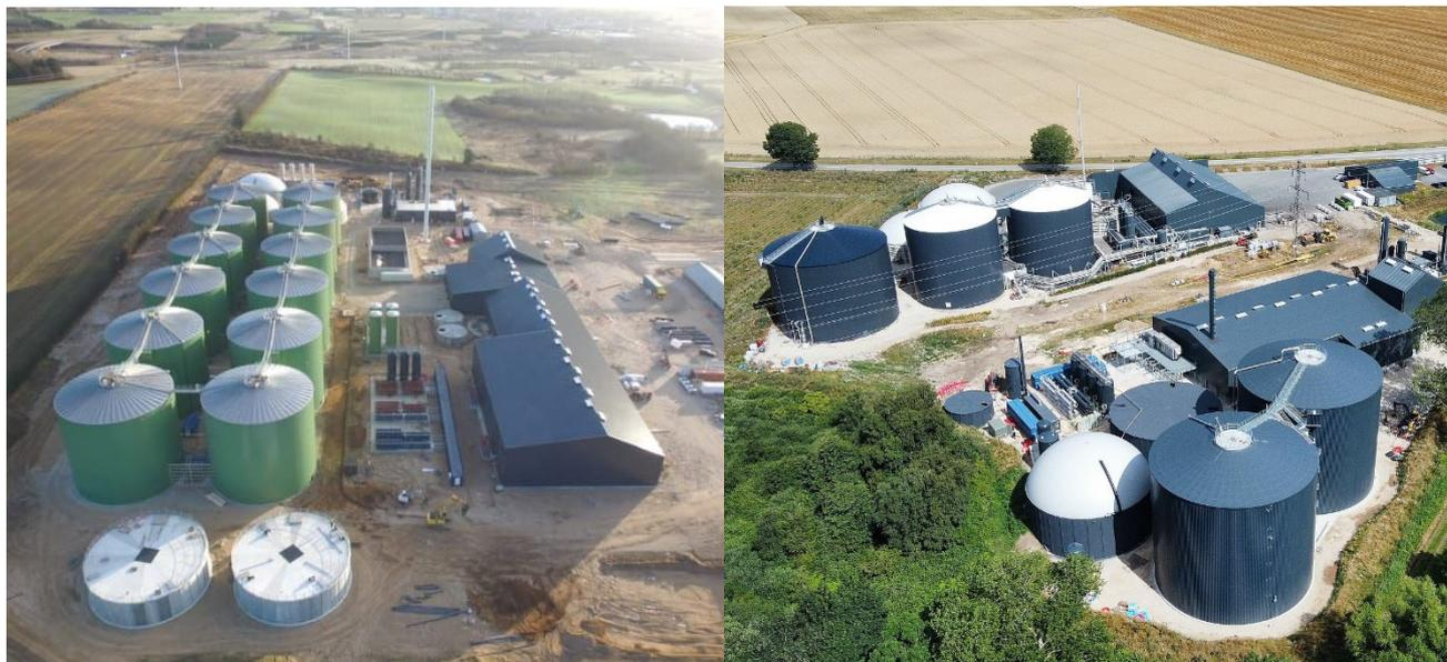
Figure 8 SBS Kliplev (to the left) is approx. 8.5 ha and has an annual production of 48 million Nm<sup>3</sup> of biomethane, whereas Solrød biogas (to the right) is approx. 2 ha and has an annual production of 11 million Nm<sup>3</sup> biomethane [23, 21]
