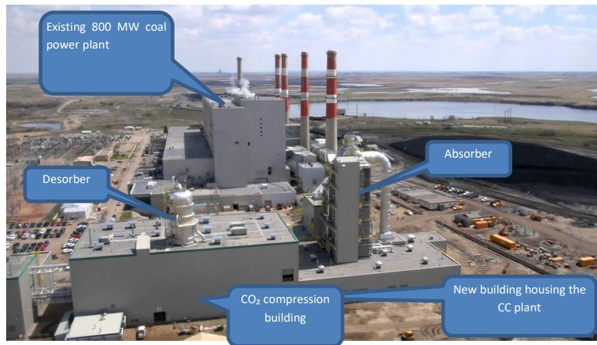
**Figure 13. Photo [37] of Saskpower 800 MW<sub>e</sub> Boundary Dam coal-fired power station where one of the four units was retrofitted with amine CC in 2013.**
