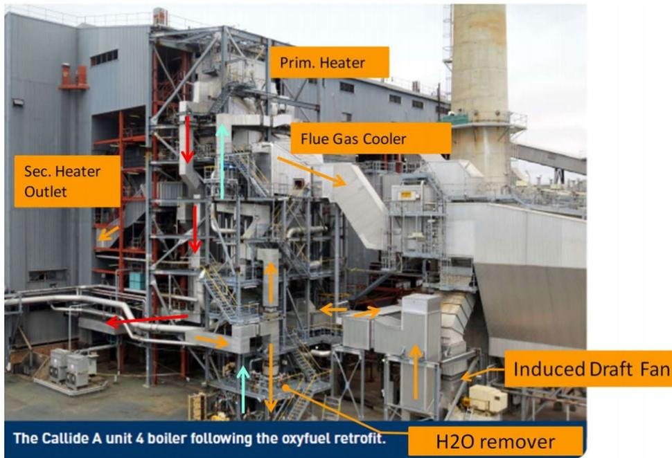
Figure 31 Photo of Callide Oxy-fuel boiler from [11] showing retrofit paths (red) and flue gas flow directions (yellow).
