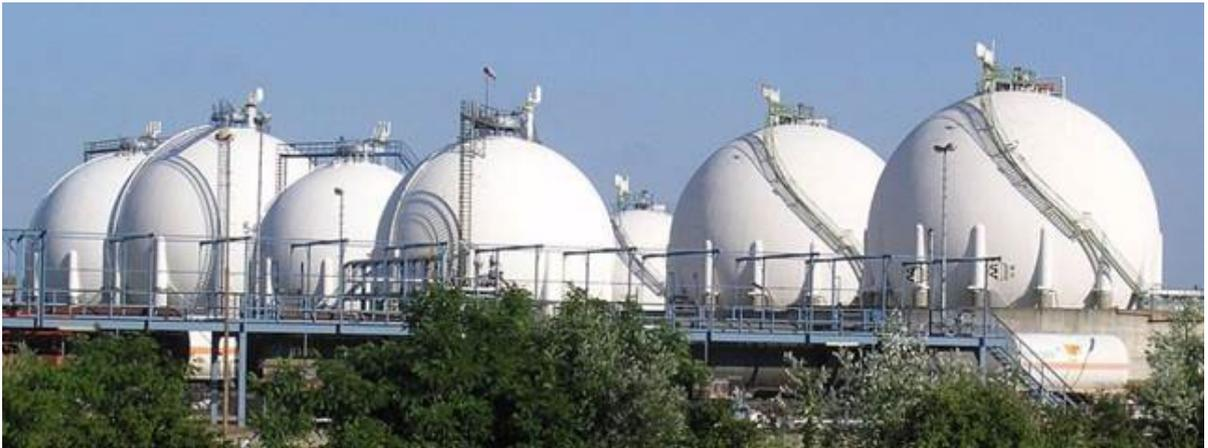
Figure 0-29: Typical gas storage tanks [21]
