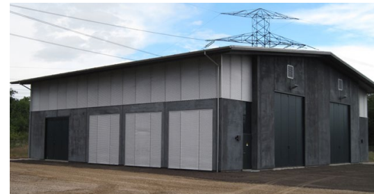
Housed 220 kV GIS
