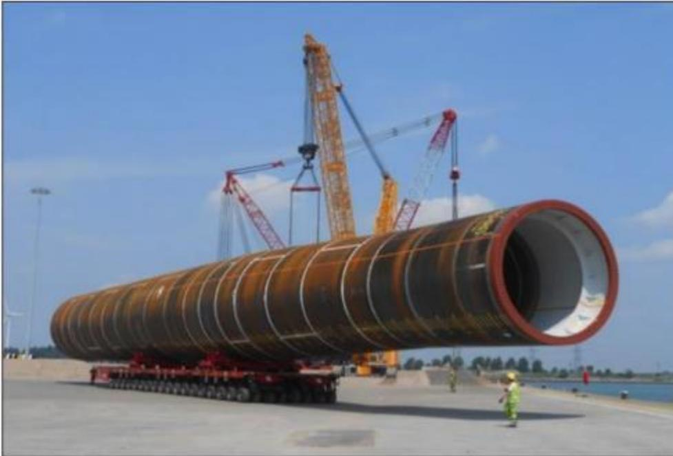
*Figure 68: Transportation of monopiles with SPMT*
