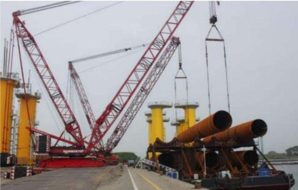
Figure 67: Loading of Monopile foundations and transition pieces
