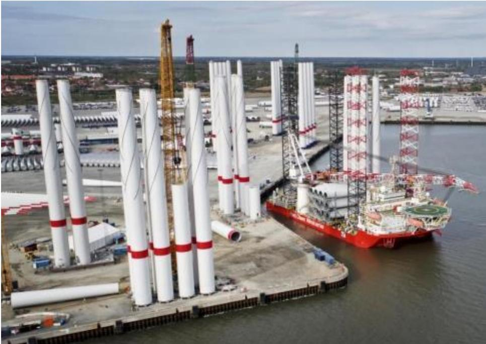
Figure 70: Tower assembly and loadout (source: Port of Esbjerg)
