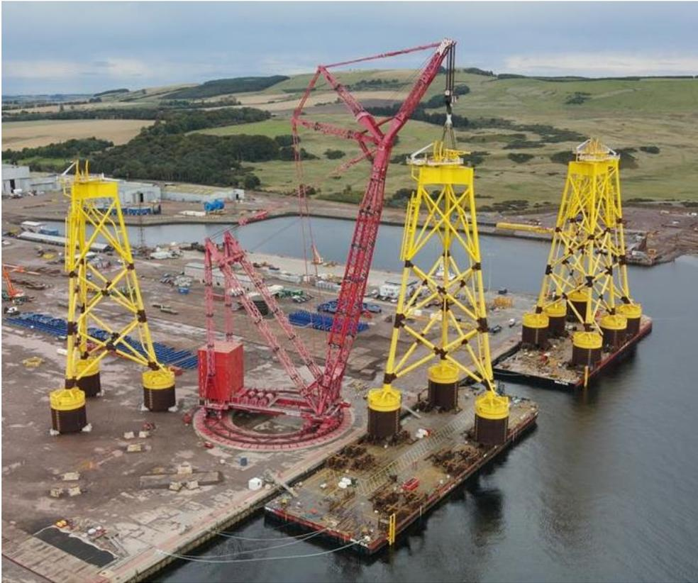
*Figure 77: Loadout of jacket foundations by ring crane. Mammoet.*
