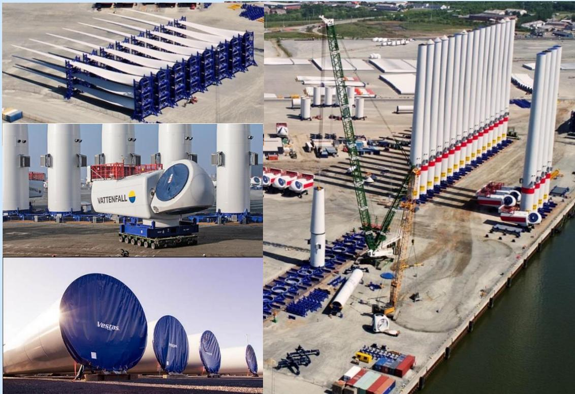
Foundation components storage, handling and transport examples
