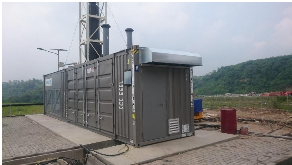
Figure 24 A containerized motor/generator system (0.8 MW) for LFG management at a landfill (Semarang, Java).
