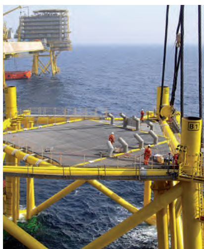
Installation of substructure for the Halfdan BD platform, 2010.
