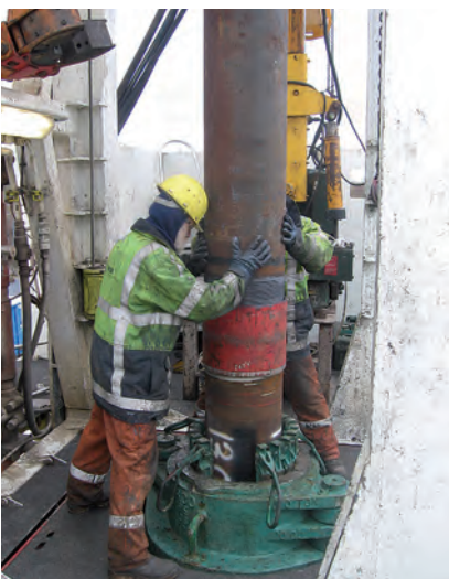
Casing is installed in well at Sønderborg.
