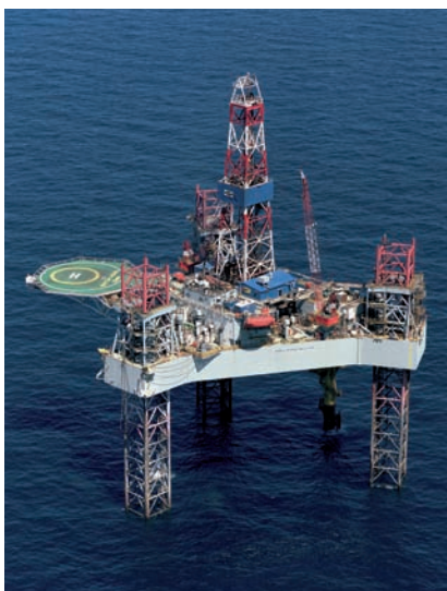
The drilling rig Nobel Byron Welliver
