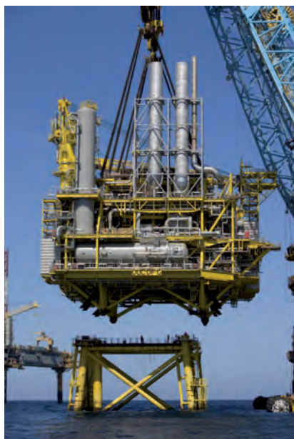
Installation of Dan FG
