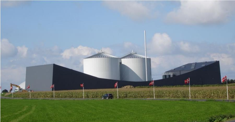
Horsens Bioenergi's co-digestion plant produces biogas from manure from local farmers and organic waste from food industries including one of Europe's largest pig slaughter houses situated very close to the plant. Horsens Bioenergi upgrades the biogas to natural gas through an upgrading plant located on the site. The plant is architecturally tailored to the landscape and the natural surroundings.
