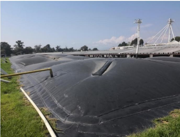
The Topoyanes Farm Wastewater Treatment Plant (WWTP) generates electric power and treated water from swine (hog) dung raised on site. The covered lagoons are built with geomembrane, liner and HDPE (High Density PolyEthylene) cover, and treat the manure from 1 000 pigs.
