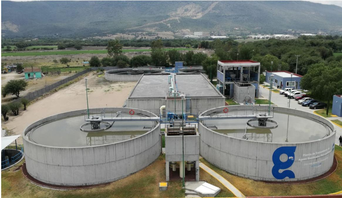
**Figure 7. Panoramic view of primary sedimentation**
