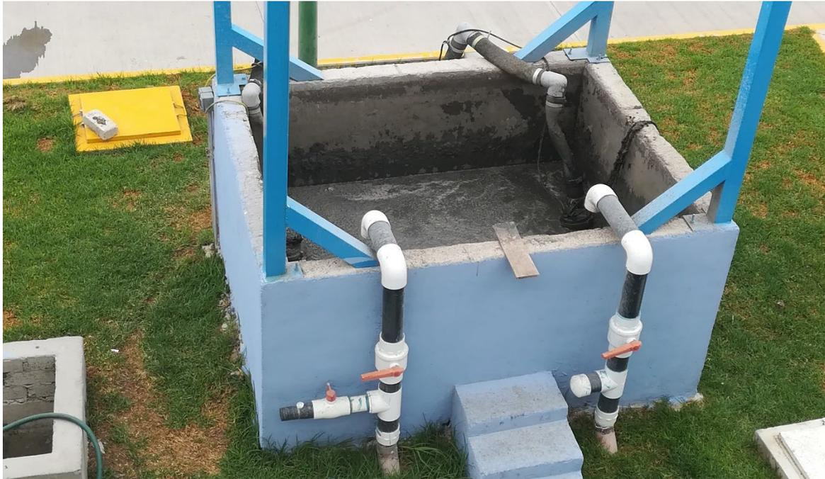
**Figure 10. Primary and secondary sludge pumping station**
