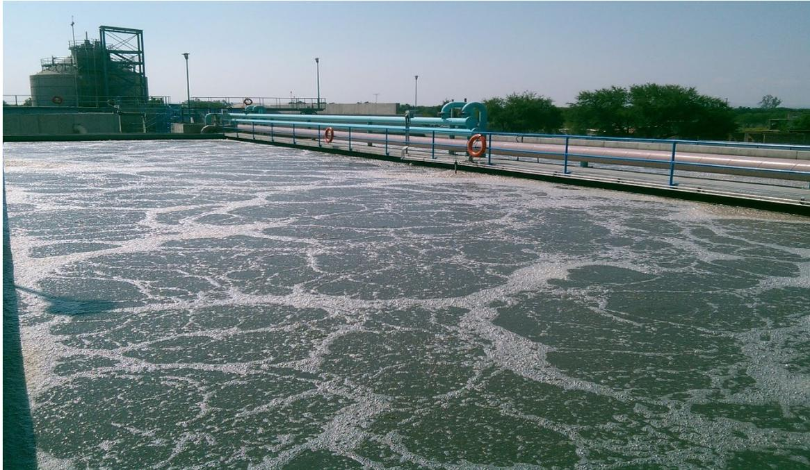
**Figure 8. Aerobic reactor**
