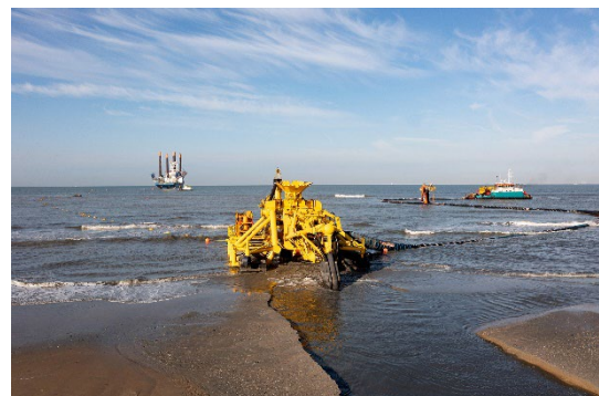
Figure 2-10 Vessel Fed Jetting
