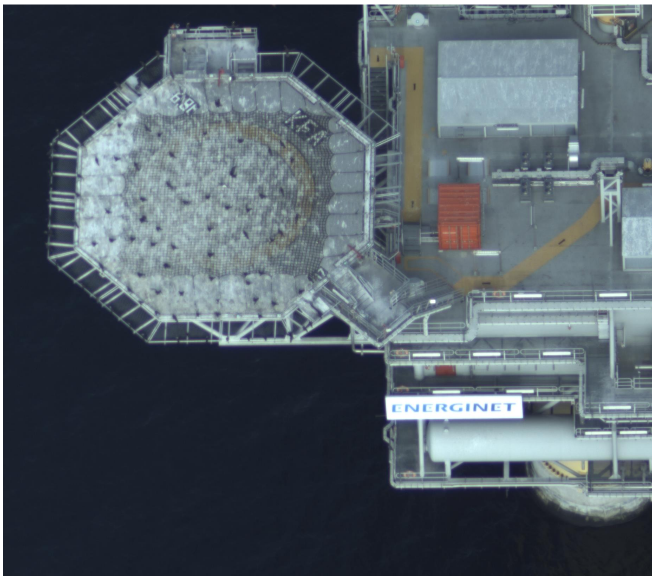
Figure 5-7 Cormorants resting on the helicopter deck of the transformer station in the OWF Kriegers Flak in February 2023.
